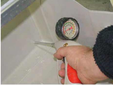
Buoyancy tank air test
